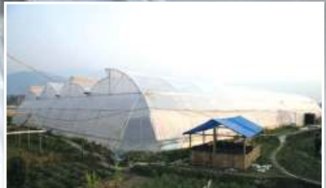
Multi Span NTS Green House
